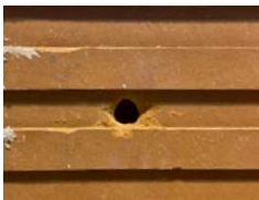
Rotary-only drilling using PYTHON spear drill bits.
