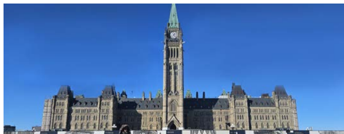
Center Block Parliament Building Retrofit.
